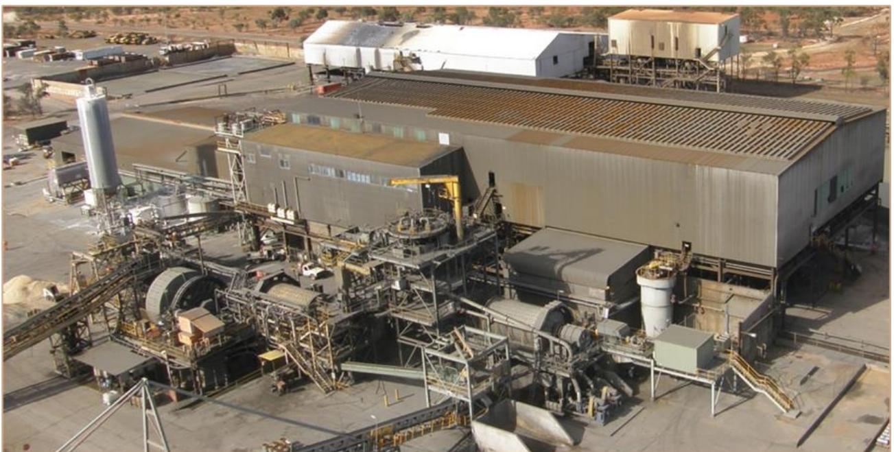
Figure 4: Endeavor Mine Processing Plant
