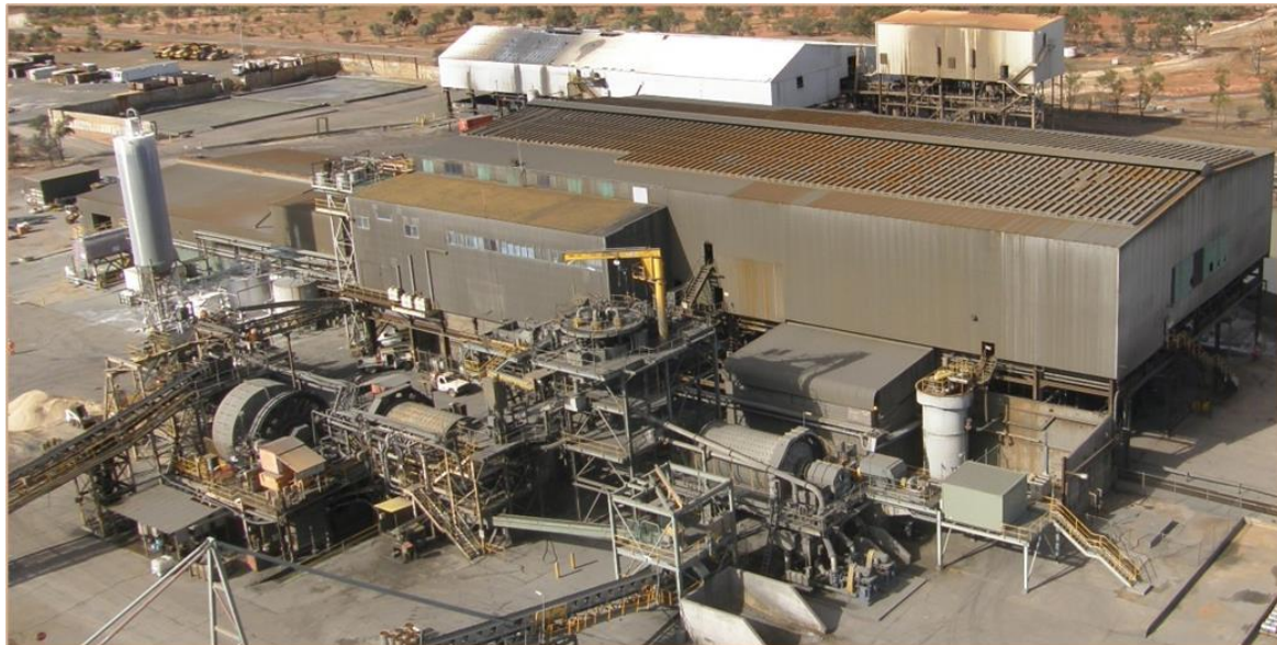
Figure 31: Endeavor Mine Processing Plant
