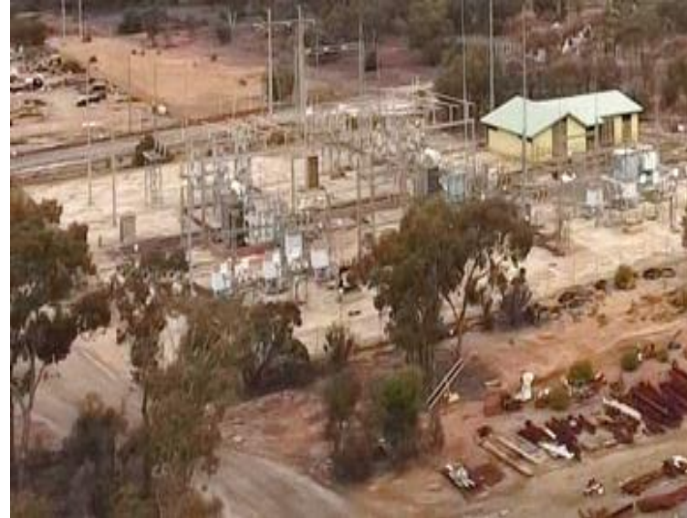
Grid power 15 MW / 132 kV, sub-station owned and maintained by Essential Energy.
