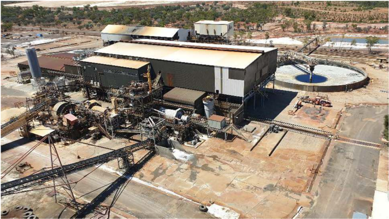
Photo 4 - Grinding, Flotation & Concentrate Areas
