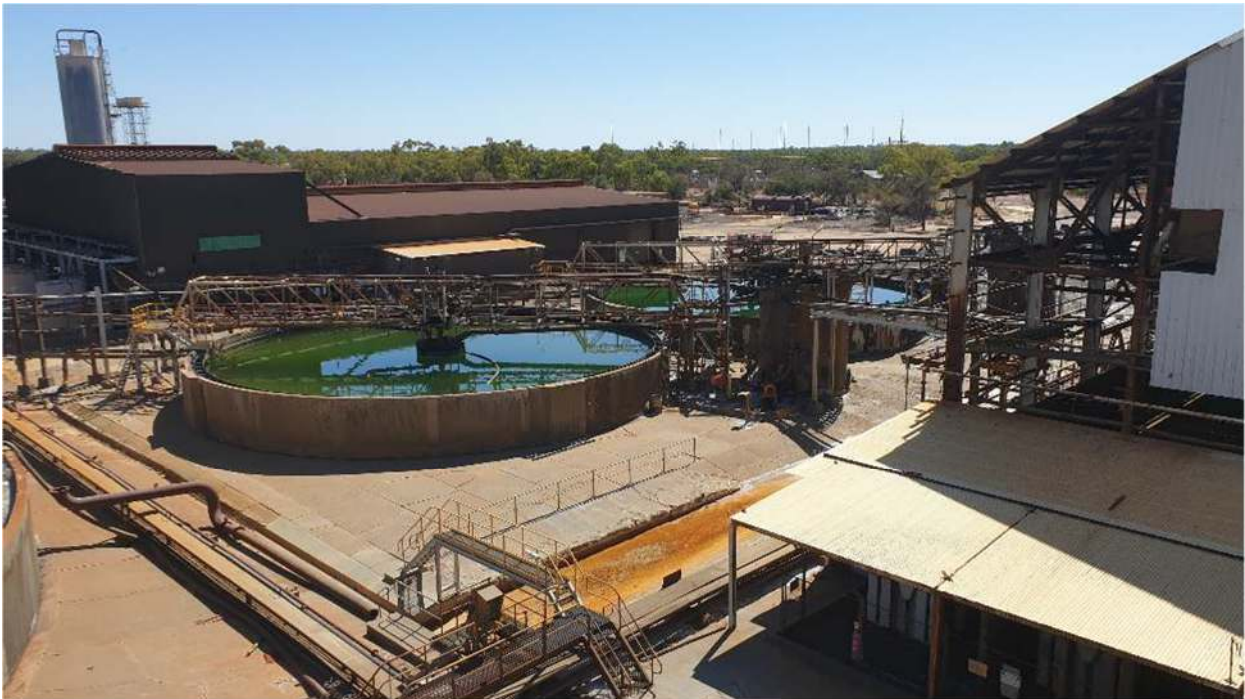
Photo 5 - Lead & Zinc Concentrates Thickeners
